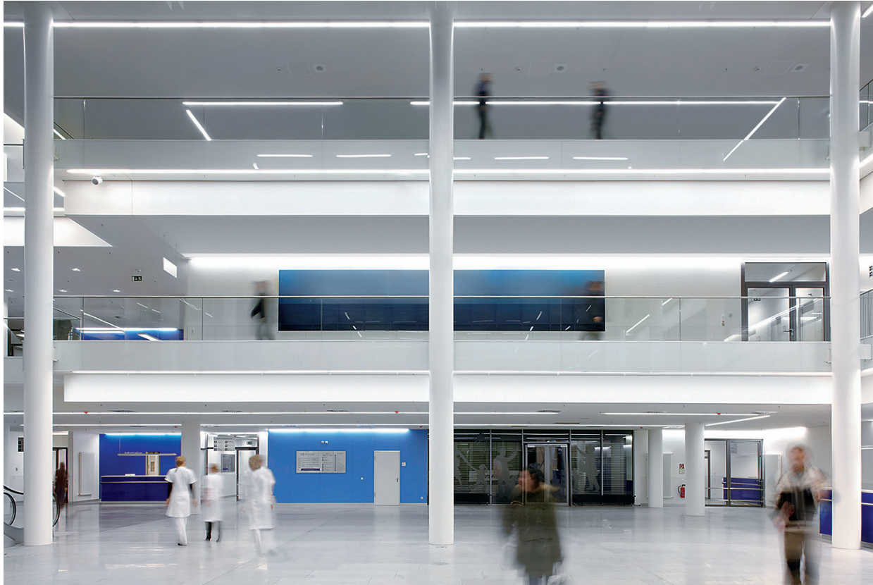
Photo: University Hospital Hamburg-Eppendorf, the new building was completed in 2008 with a lighting solution by the Zumtobel Group, first request for an upgrade to LED in 2018, Step 1 was a refurbishment solution with 2 km Slotlight Refurbishments Kits and new TECTON LED inserts in the entrance hall, Step 2 Refurbishment Kits for CLEAN in the operating theatre anteroom, airlocks and intensive care areas, Step 3 Refurbishment solution for lecture theatre with Panos Planned completion August 2022.
